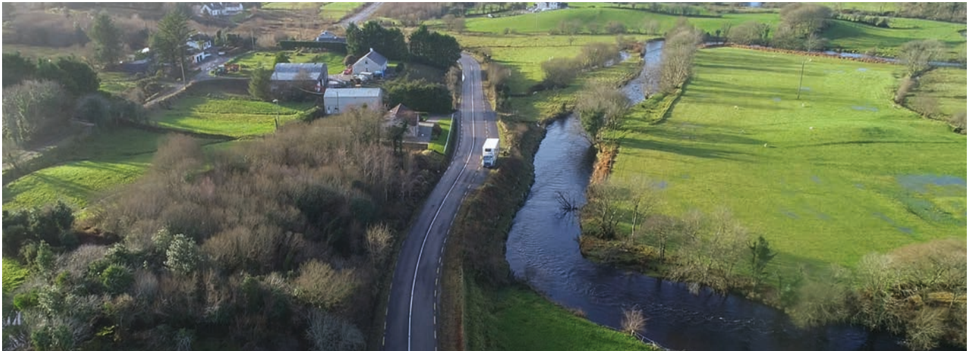
The N56 road running alongside the environmentally sensitive Owenea River which is home to the Freshwater Pearl Mussel.
