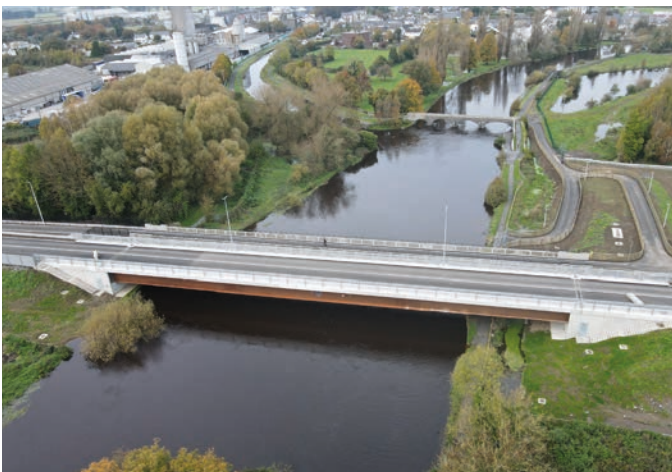
The new 80m single-span steel composite road bridge crossing the river barrow.
