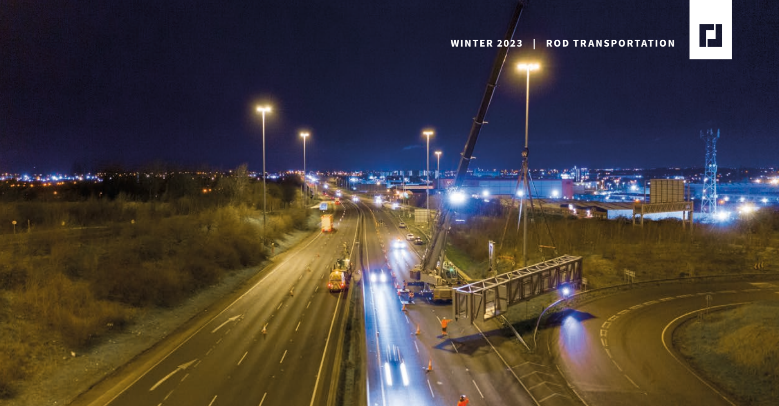
Gantry installation at Junction 9 Red Cow.
