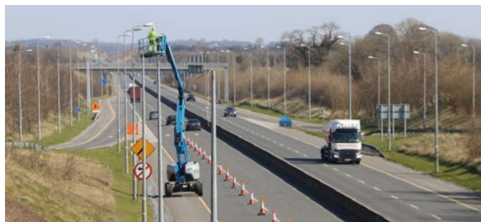
Lighting Column Removal on the M6.
