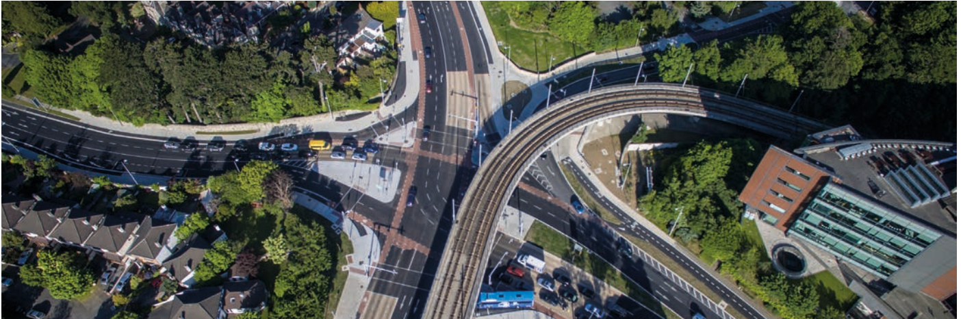
Leopardstown Junction Upgrade, Sandyford.
