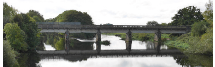
The refurbished existing railway bridge now caters for pedestrian and cycleway traffic over the river Barrow.
