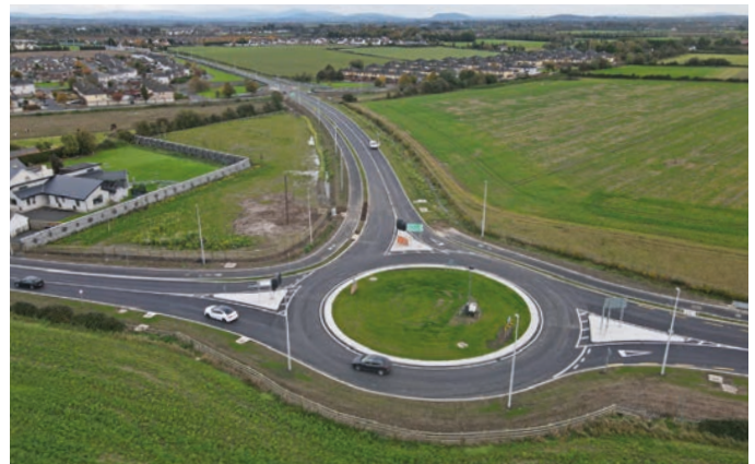
The new N78 roundabout at the southern end of the scheme.
