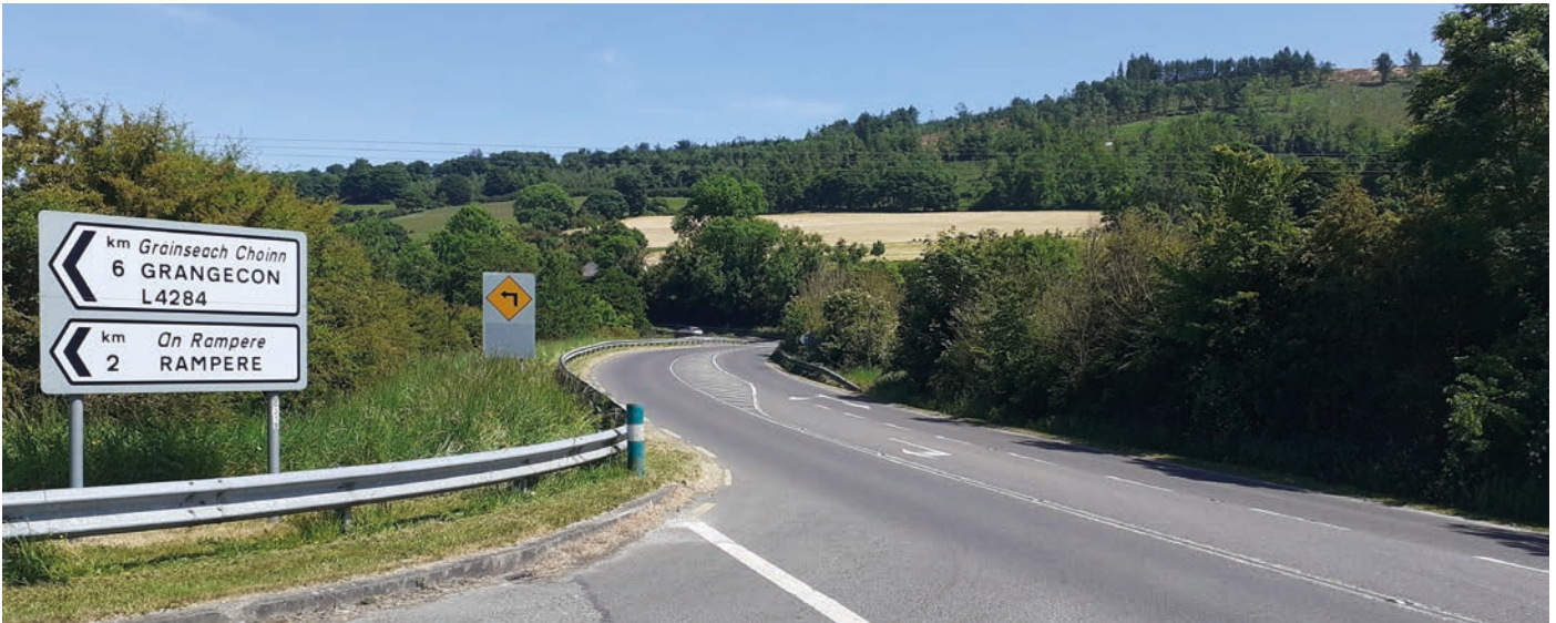
N81 Eldon Bridge Bends, Tuckmill Upper.
